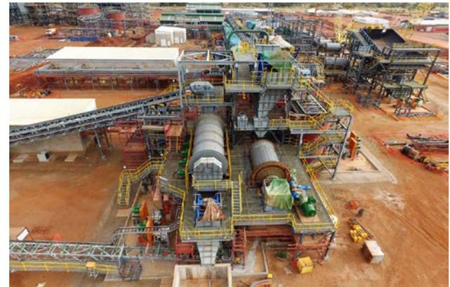
*Ore bin (top) and primary mill and flotation (bottom)*
