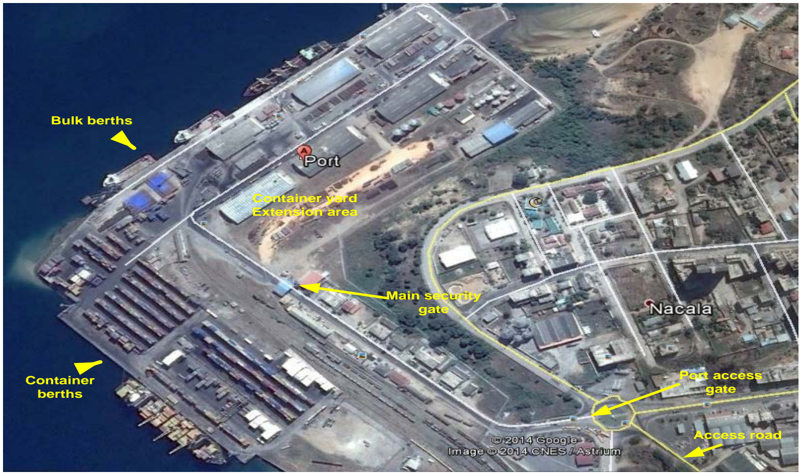
Area view of the Port of Nacala
