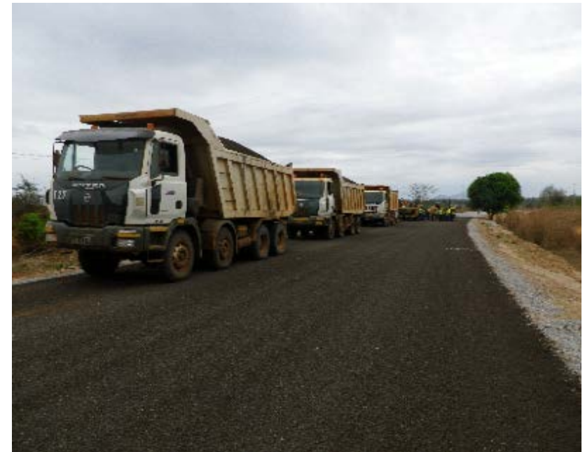
Newly completed bitumen road
